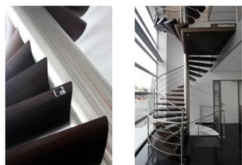
Left: Close-up of the staircase pivot with the invisible tread suspension system
